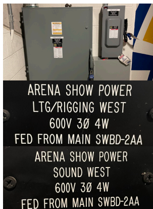
3rd Floor NW Corner
