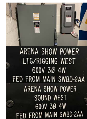
3rd Floor NW Corner
