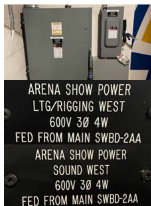
3rd Floor NW Corner
